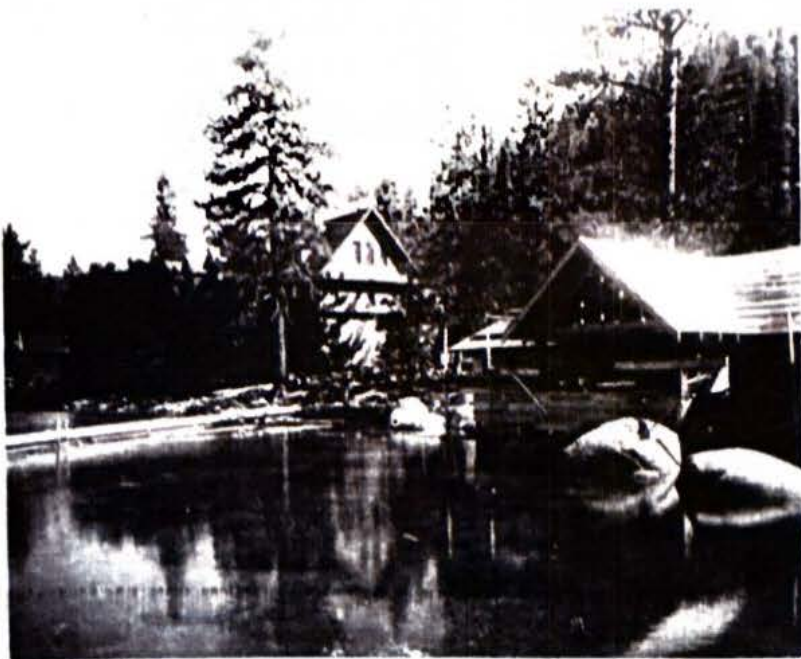
Bath house under construction next to the Brockway Hotel on the left. Lake Tahoe Photographic Shore Line Survey, July 19, 1916.
