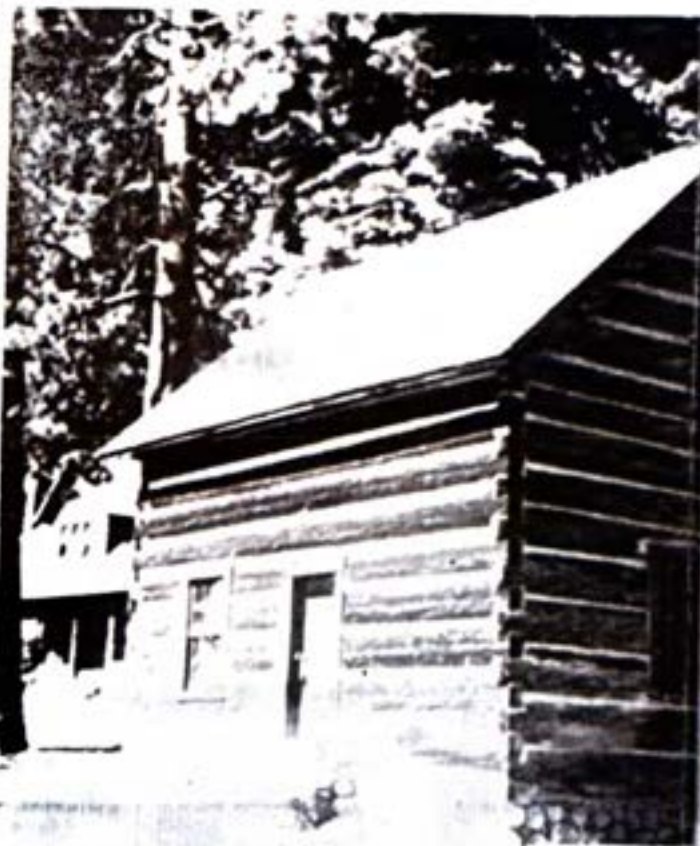
Built in 1870, the General Phipps Cabin, located at Sugar Pine Point State Park, is still standing on the West Shore.
