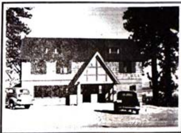
Tahoe City's newly-completed Community Center, on the bluff above Commons Beach, awaits occupancy in June, 1938. (C.W. Vernon photo courtesy of Lillian Vernon Farr)
